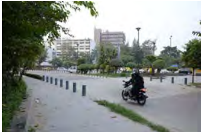
Figure 55. Speed table doubling up as a mid-block crossing with safety bollards in New Delhi, India. (Source: The World Bank)
