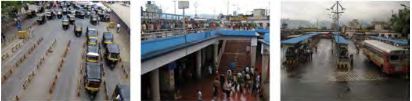
Figure 70. Thane Suburban station in India with lower level for auto-rickshaws and upper levels for bus bays. It connects to the road level via elevated walkways (Source: WRI India)
