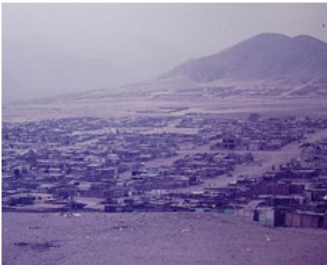
Figure 4-1: Overview of the Villa El Salvador slum, 1975. (Source: Institute for Housing and Urban Development Studies 22 )
