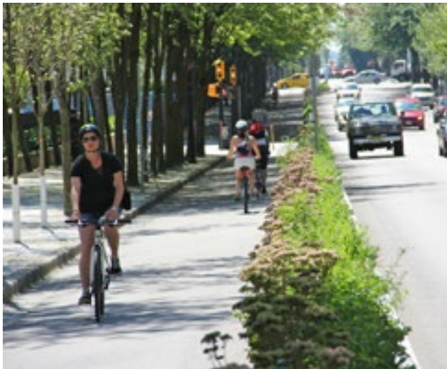
Figure P7-19: A one-way, dedicated bike lane offers protection from the street and sidewalk by using tree buffers. (Source: Paul Krueger, CC BY-SA 2.0, https://commons.wikimedia.org/wiki/File:Hornby_Street_Separated_Bike_Lane.jpg )
