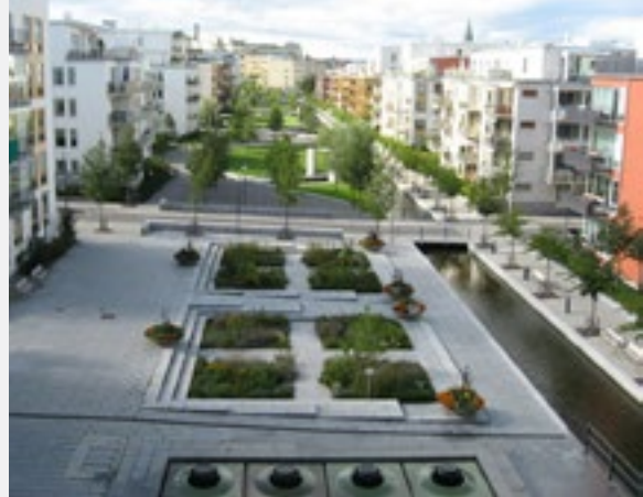
Figure P6-44: Water canal and floodable plazas (Source: Design for Health/Flickr, CC BY 2.0, https://www.flickr.com/photos/designforhealth/6359946395 )
