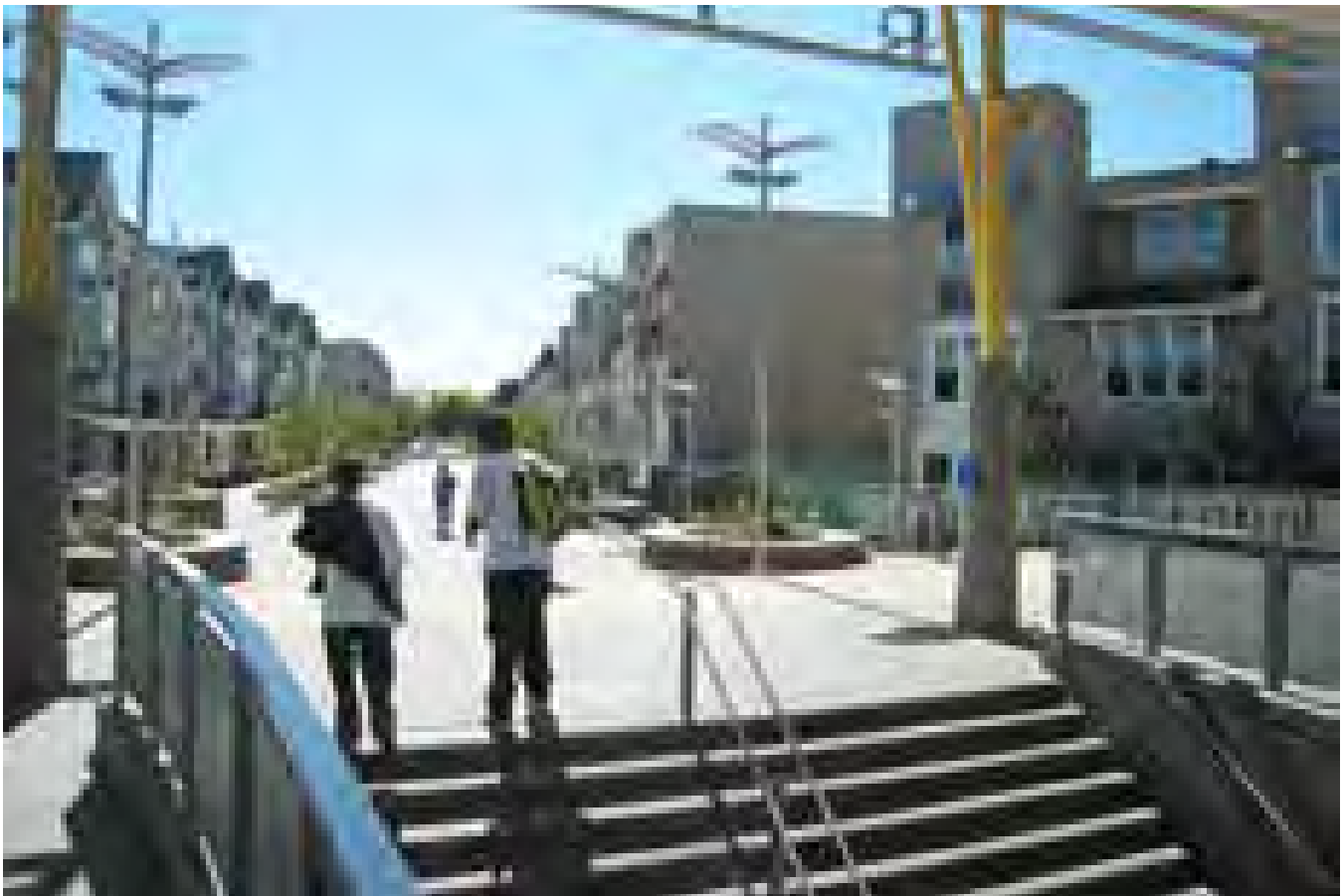
Figure P4-10: Richmond Transit Village is a transit-oriented development that includes mixed-ownership and mixed-income housing situated around BART's multimodal transit station in Richmond, California. A wide pedestrian promenade running between the station's grand entrance and the village provides direct access to transit. (Source: HDR | Calthorpe)
