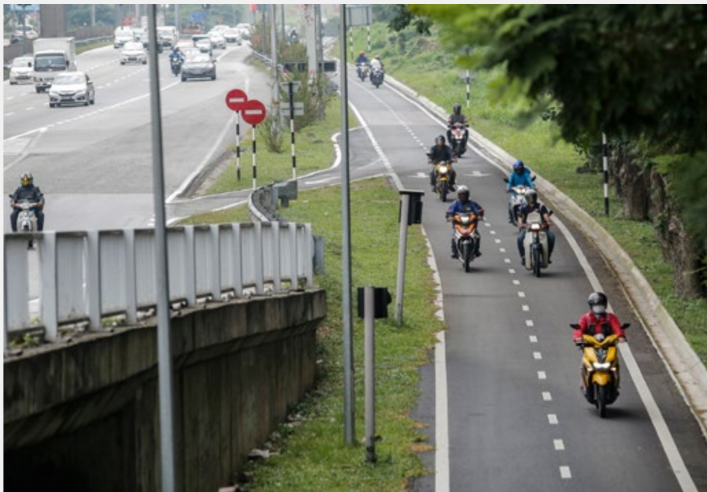
Figure P3-20: Separated, dedicated motorcycle lane along one of Malaysia's highways. (Source: Shutterstock)
