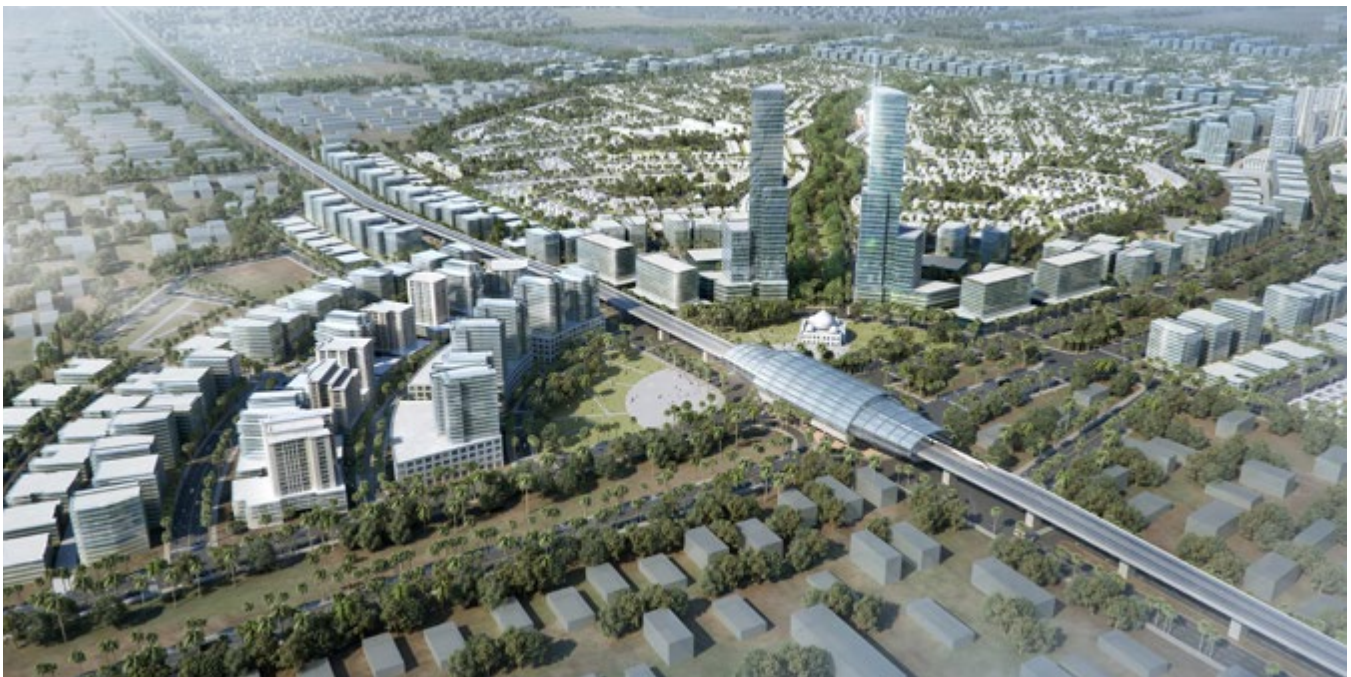
Figure P3-8: The Al Rabwa mixed-use development located in central Riyadh, Saudi Arabia offers a sustainable approach to providing a variety of residential and commercial uses with transit accessible destinations and walkable neighborhoods. (Source: HDR | Calthorpe)
