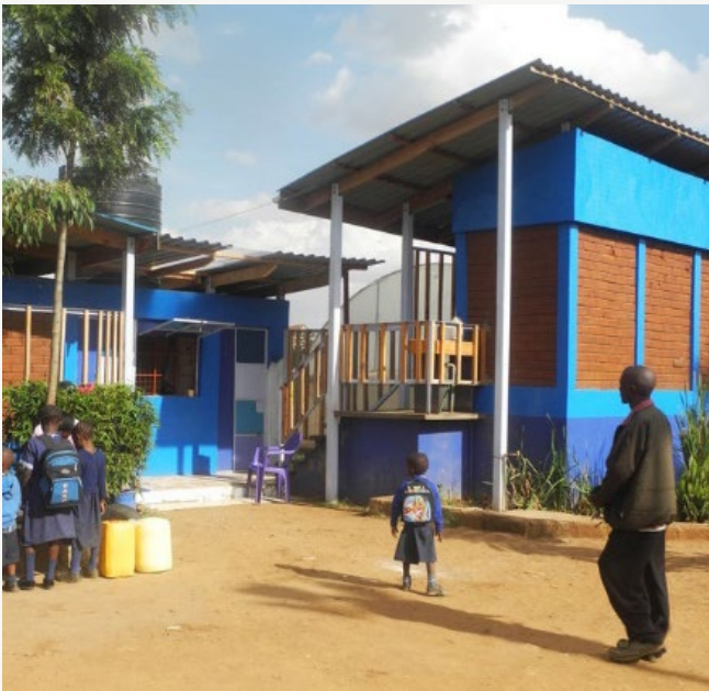
Figure P2-3: This KPSP site includes a public sanitation block with rainwater capture to irrigate crops, waste collection, and composting for floriculture operations. (Source: KDI)
