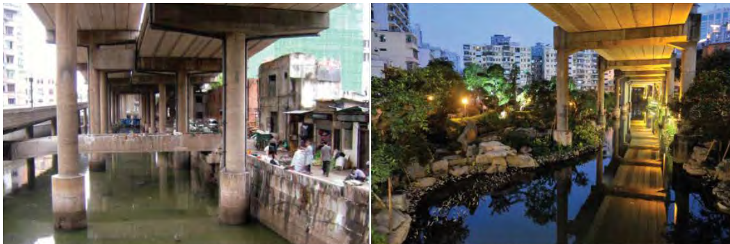
Figure 24: The Donghaochong Canal before and after restoration efforts to improve the vital public space along the BRT corridor. | Source: Far East BRT Planning Co., Limited ©Far East BRT Planning Co. Reproduced with permission from Far East BRT Planning Co.; further permission required for reuse.
