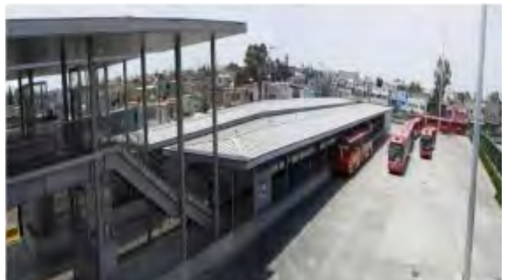
Tepalcates Central Station (After)
