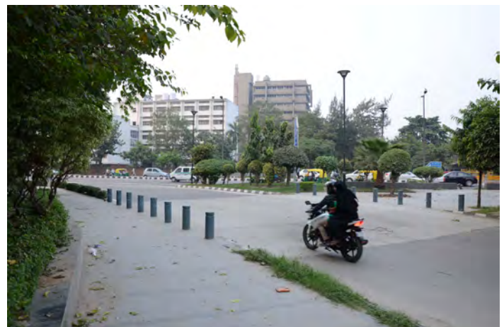
Figure 55. Speed table doubling up as a mid-block crossing with safety bollards in New Delhi, India. (Source: The World Bank)
