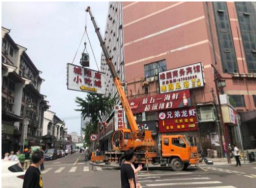
Figure 4: Renovating Facades on Kaiming Street
