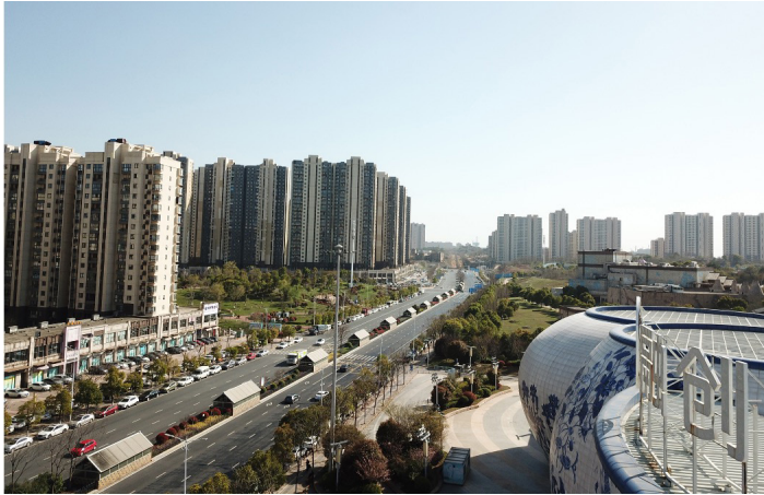
Figure 5: Commercial Integration at Jiulonghu Lake South Station
