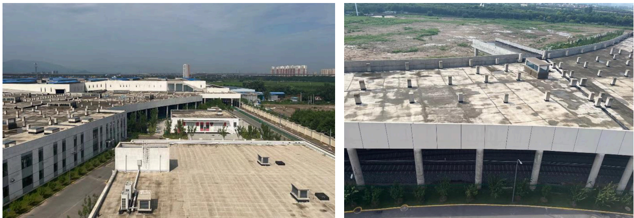
Figure 7: Current Situation of Overhead Development at Jiahua Depot
