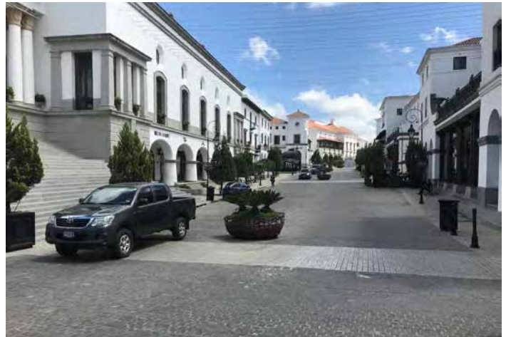
Shared street in Guatemala with different material, bollards and planters to reduce speeds of moving vehicles, creating safer space for other road users. (Source: © The World Bank)
