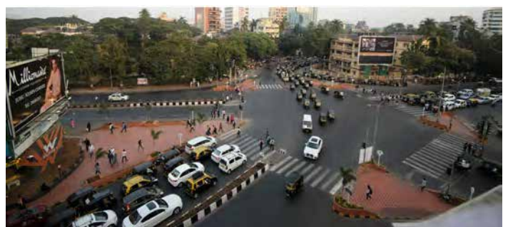
Slip lanes provided as part of HP Intersection redesign in Mumbai, India
