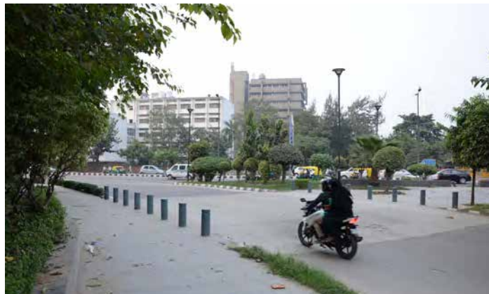
Speed table doubling up as a mid-block crossing with safety bollards in New Delhi, India (Source: © The World Bank)
