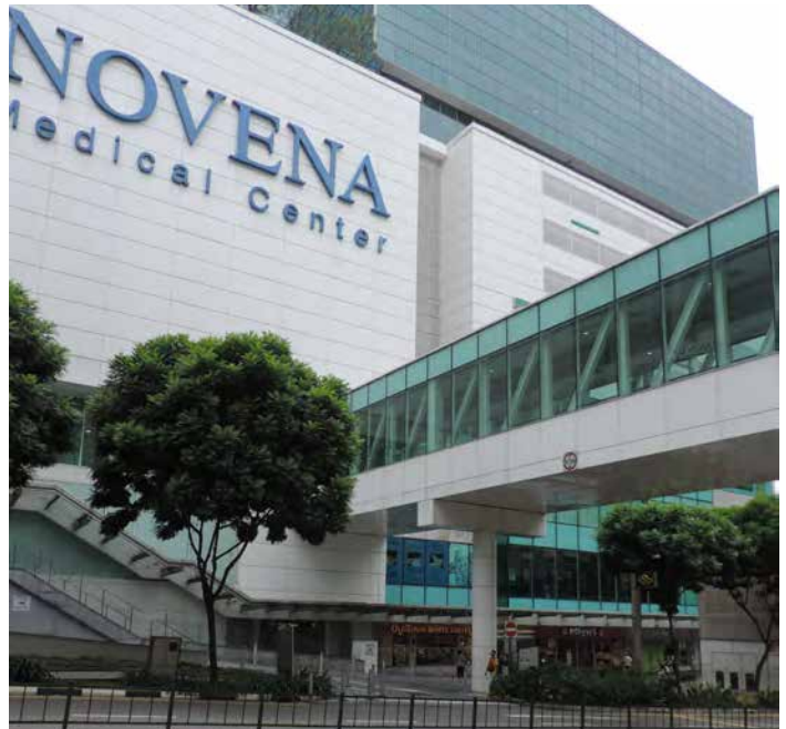
Foot-over-bridge connecting to the mixed development at the Novena MRT Station, Singapore (Source: © The World Bank)
