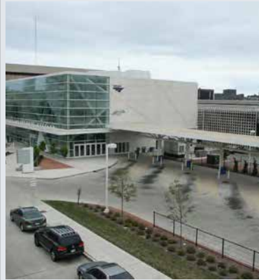
Milwaukee Intermodal Station
