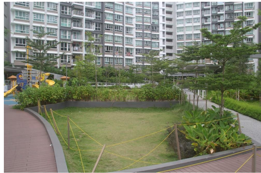
Rain garden and bioretention basin in residential estate for stormwater management (Tan Puay Yok)
