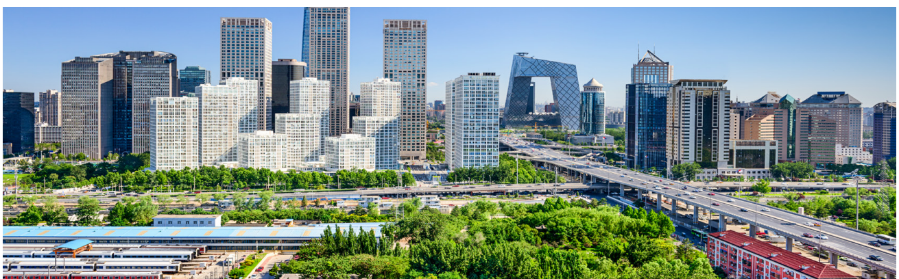
Urban green and grey infrastructure in Beijing, China
