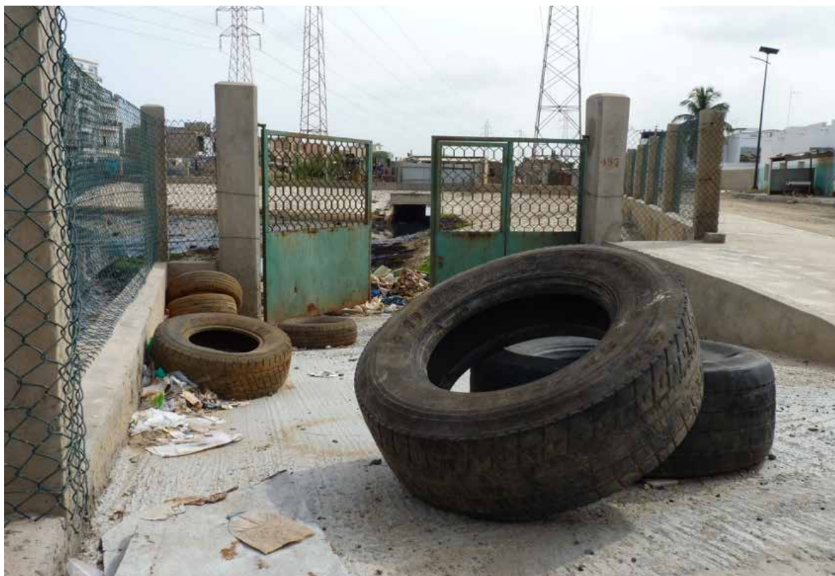
Without maintenance and care, the works carried out are exposed to the risk of rapid deterioration. In the photo, waste accumulation at the entrance to the Dalifort-Foirail retention pond.
