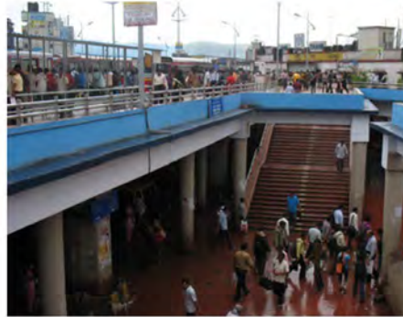
Thane Suburban station in India with lower level for auto-rickshaws and upper levels for bus bays. It connects to the road level via elevated walkways (Source: © WRI India)
