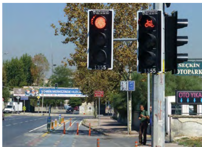
A bicycle signal is provided along a protected bicycle lane in Istanbul, Turkey (Source: © WRI)
