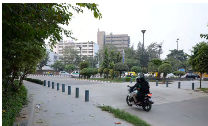
Speed table doubling up as a mid-block crossing with safety bollards in New Delhi, India
