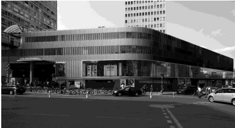
Gare Montparnasse, the renovated façade, 2020
