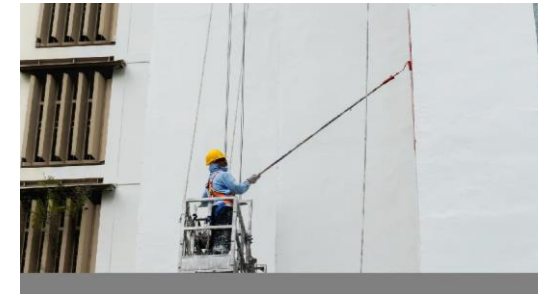
Materials (cool paints, permeable surface)
