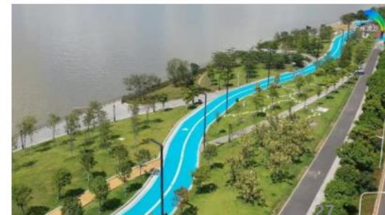
The Dyke of Nansha Bay
