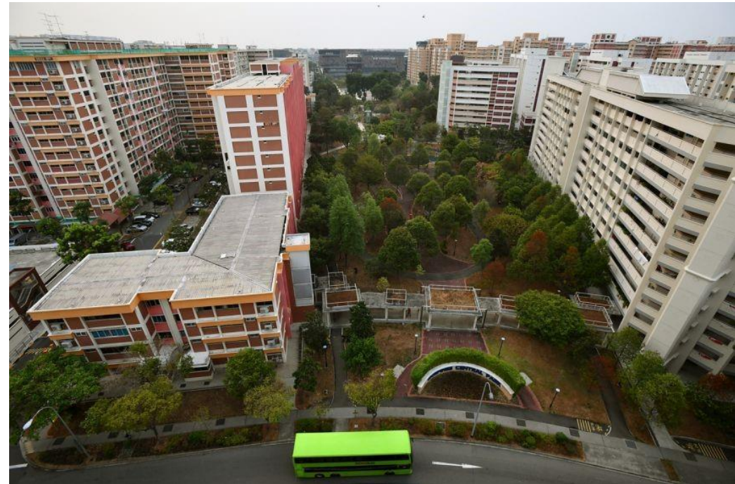
Large-scale pilot project at 130 blocks in Tampines
